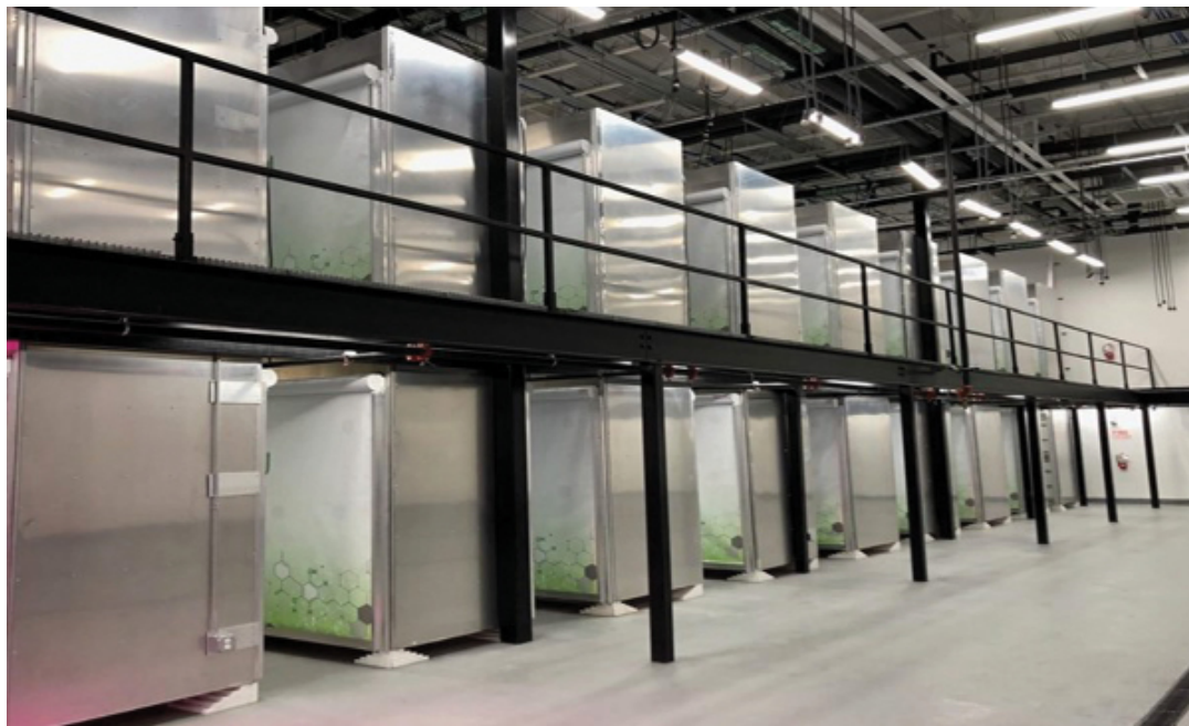
Facility with AVFUs
