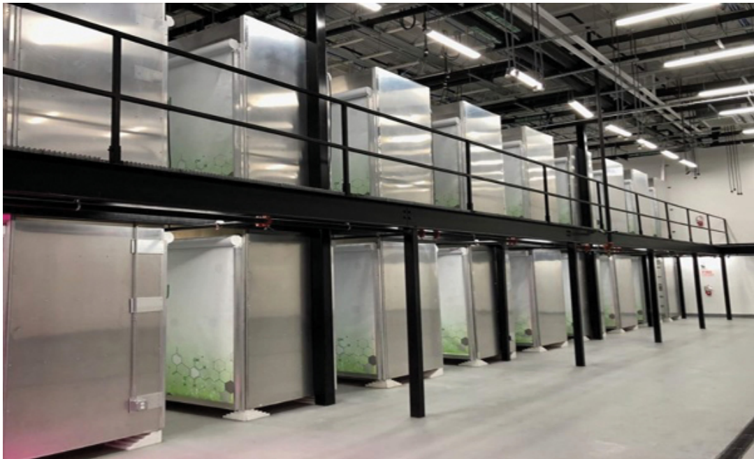
Facility with AVFUs
